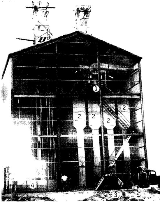
Figure 19-9. A column-type rice drier: (1) cleaning machinery, (2) columns, (3) dump pit, and (4) hot-air fans.
