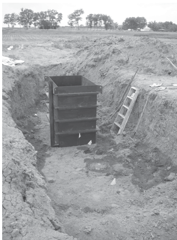
FIGURE 5.18 Installation of a lysimeter at St. Joseph Research Station, St. Joseph, Louisiana.
