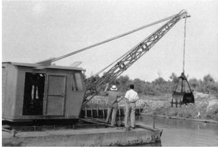
Fig. 6.15 Dragline excavator, operated from pontoons in tidal lagoons in Italy, for dike construction. (Photograph: Carlo Mozzi.)
