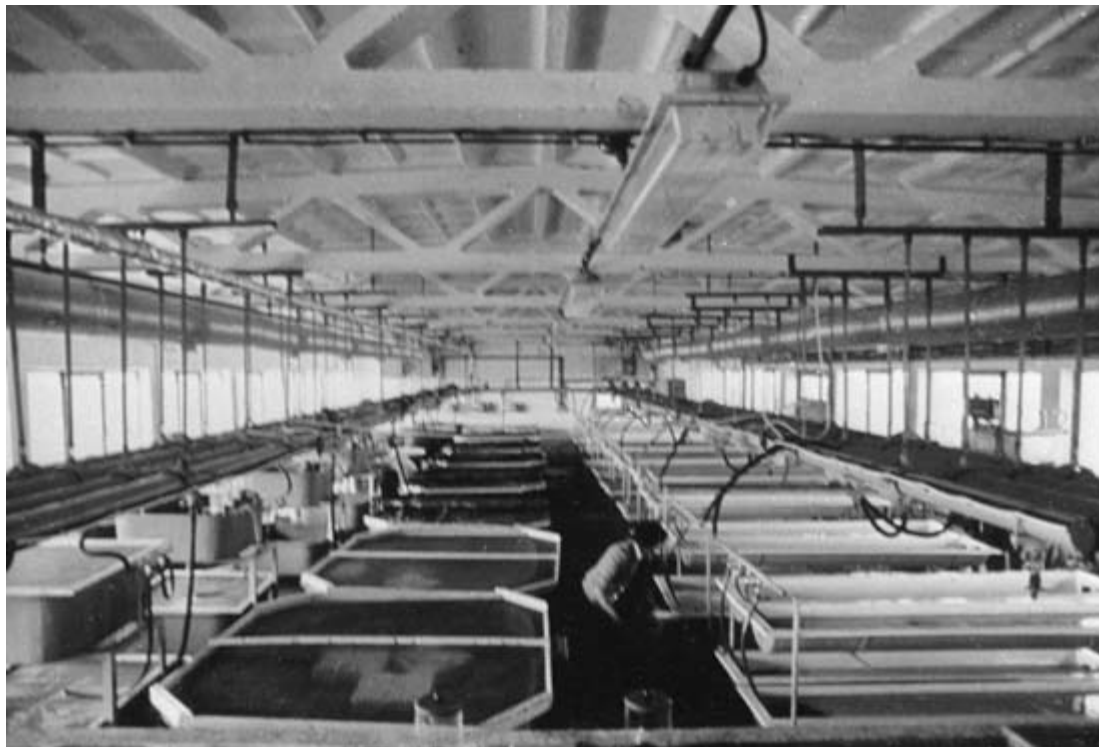
Fig. 6.40 Troughs made of fibreglass and aluminium used in a modern carp hatchery in Hungary.
