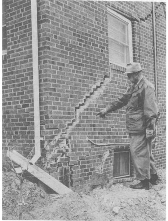
**FIGURE 3.5** Foundation soil with high clay content expanded and shrunk with wetting and drying, cracking the wall. (Photograph courtesy USDA.)
