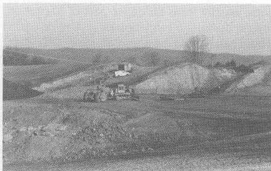
**FIGURE 19.5** Sites selected for solid waste disposal (landfills) need water-impermeable underlying strata to minimize groundwater pollution.
