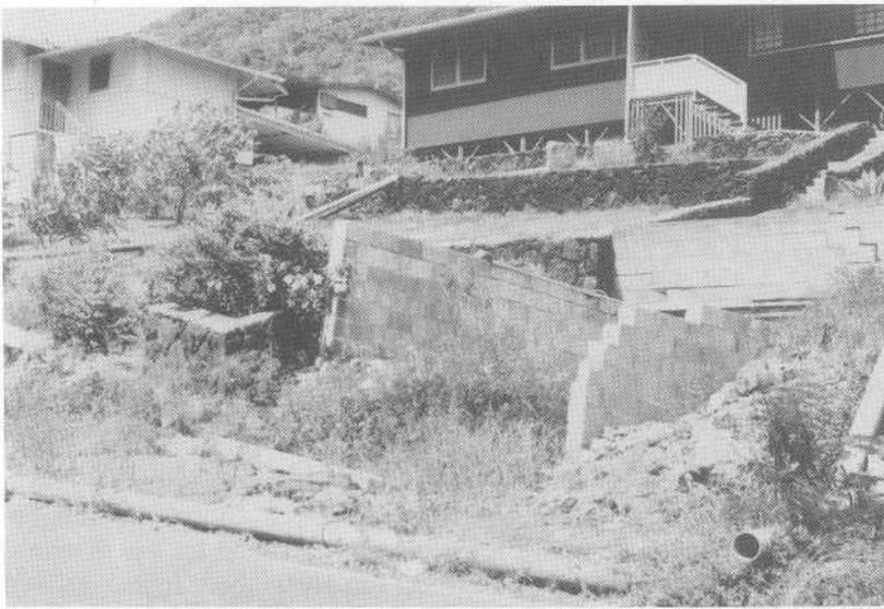
**FIGURE 18.28** Structural failure caused by landslide on Vertisols produced by wet soil sliding downhill. Note that pipes are on top of the ground to prevent breaking caused by expansion and contraction of soil.
