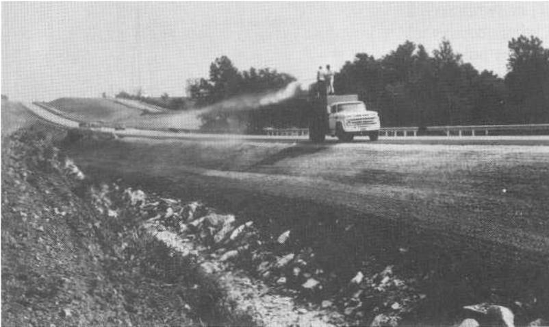
**FIGURE 7.11** Slurry truck spraying fertilizer and seed on freshly prepared seedbed along road in Missouri. A thin layer of straw mulch will be secured with a thin spray of tar to protect the soil until vegetation becomes established. (Photograph courtesy Soil Conservation Service, USDA.)
